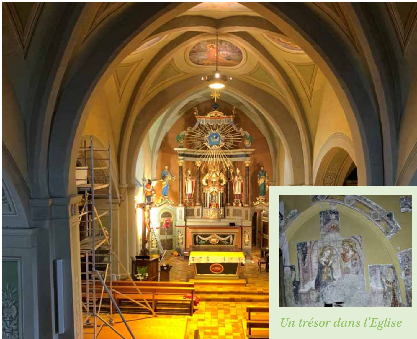
photo : In Situ Conservation
